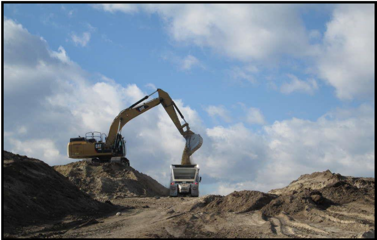
Figure 4.10 – Four Mile Drive Construction
