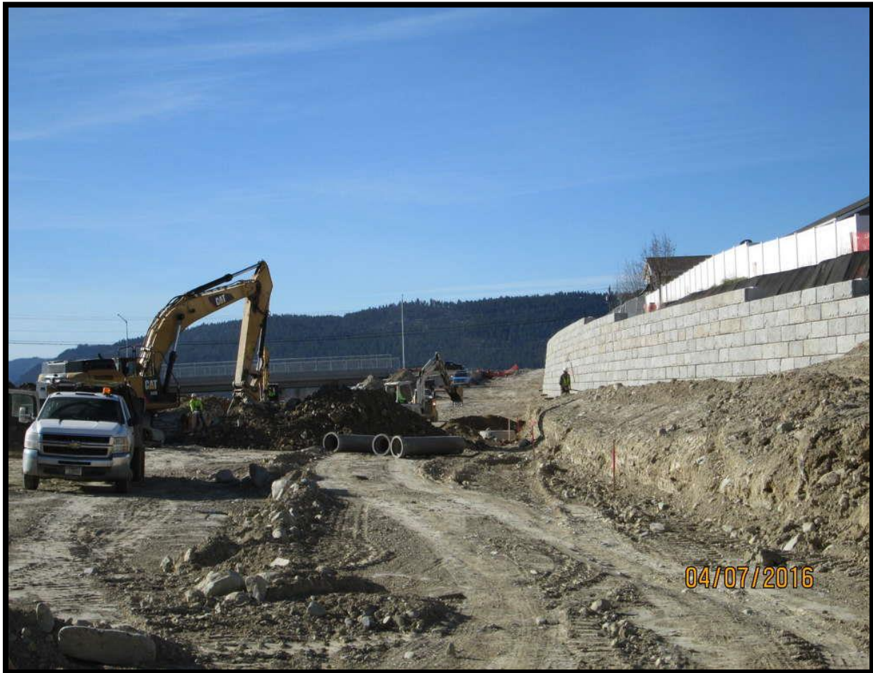
Figure 2.4 – Retaining Wall Construction by Empire Estates
