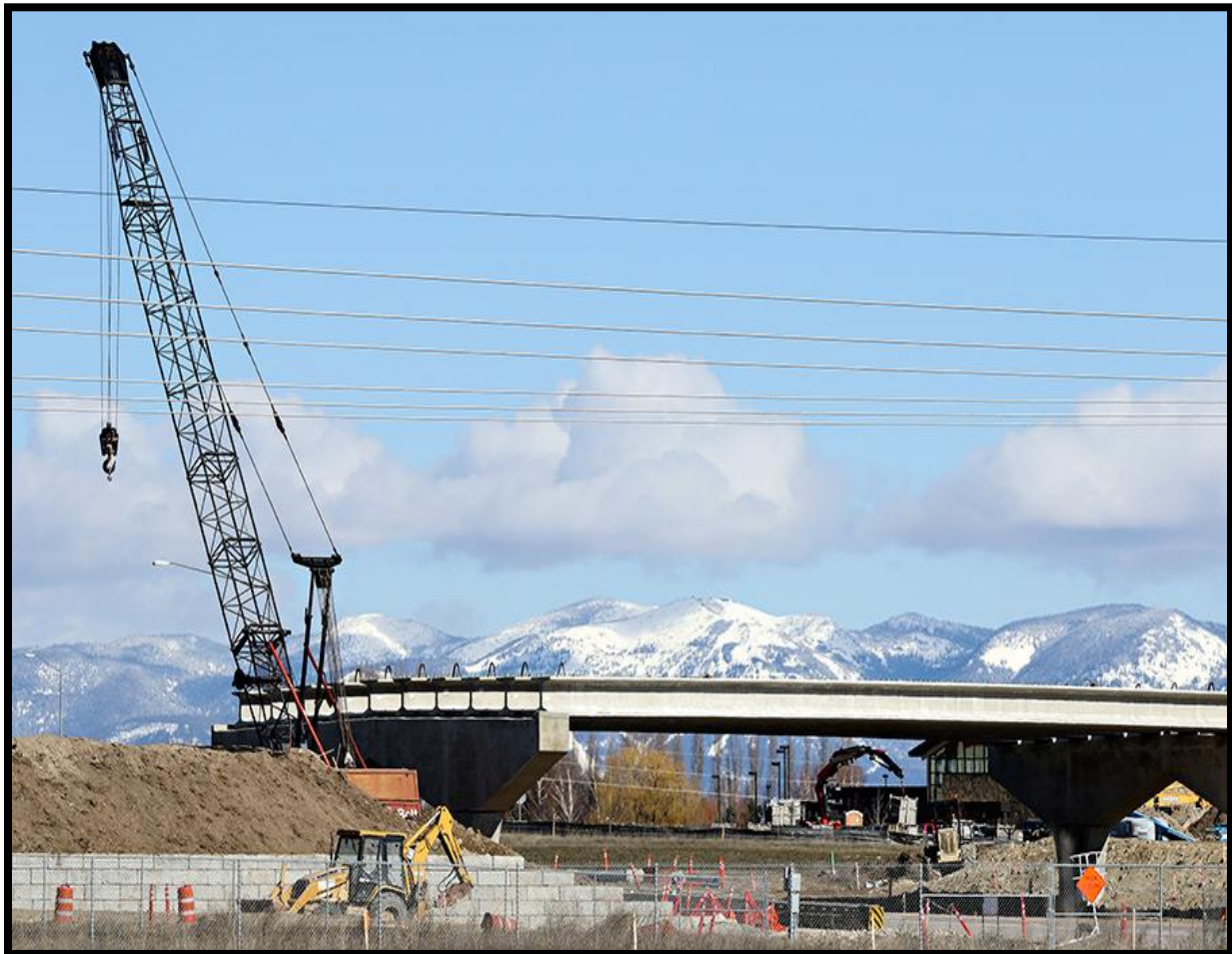
Figure 2.3 – Construction of the Old West Reserve Bridge by Glacier High School
