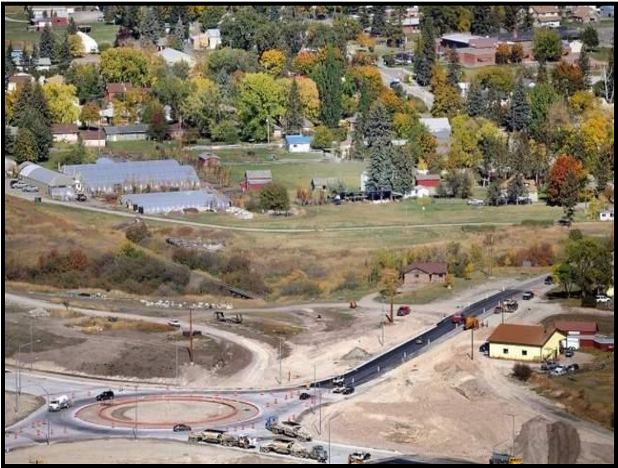
Figure 1.6 – Foy's Lake Roundabout Construction in 2010
