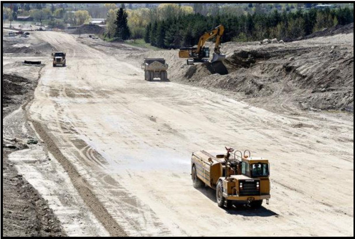
Figure 2.2 – Bypass Construction South of Three Mile Drive
