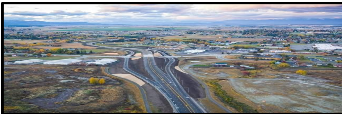
Figure 4 – Bypass Interchange at US 2
