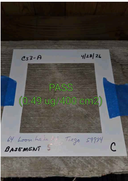
CS3 A - Basement 5, Beam
