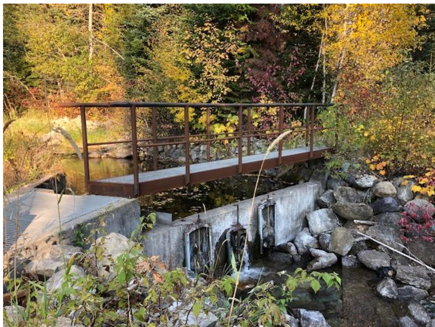
The Second Creek diversion dam. The water is backed up behind it to the left.
