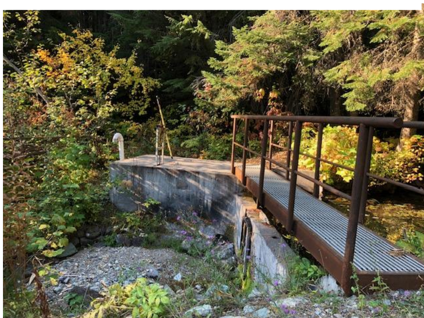
The Third Creek diversion dam. The water is backed up behind it to the right
